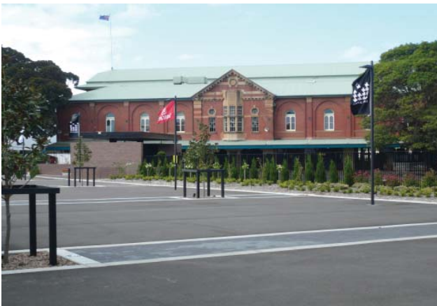
Figure 3.10 The rear of the Members' Stand, shown above, is on the eastern boundary of the subject site
