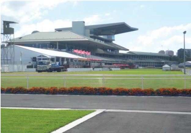
Figure 3.15 View along the eastern boundary of the Spectator Precinct showing the Marque, Paddock, Queen Elizabeth II and Member's Stands
